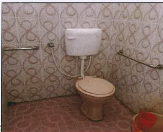
TOILETS WITH HAND RAILS
